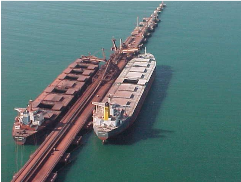
Figure 2: Iron Ore Terminal (Saldanha & Langebaan Side)
